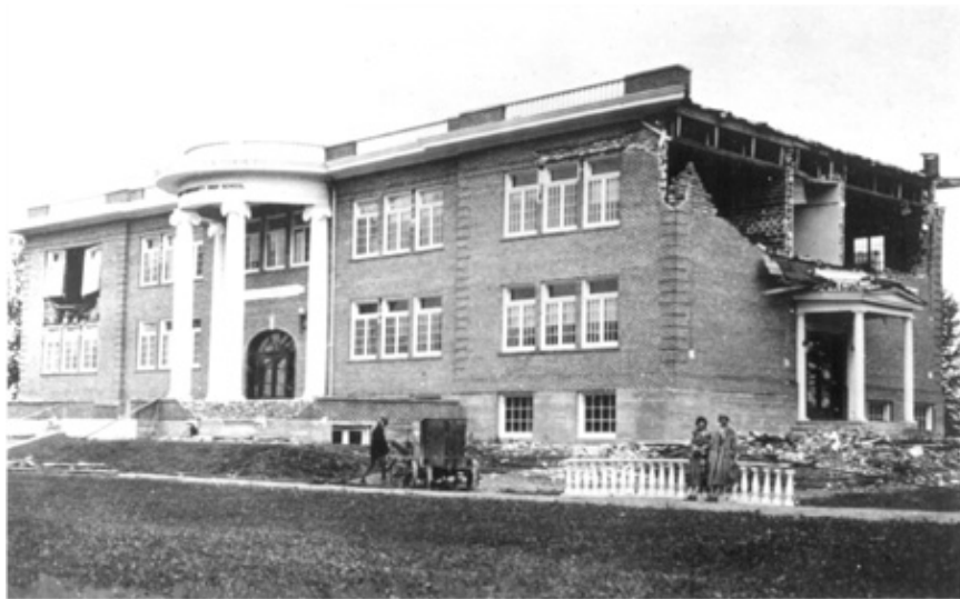
Figure 4.3.2: Damage to Community High School at Manhattan, MT
