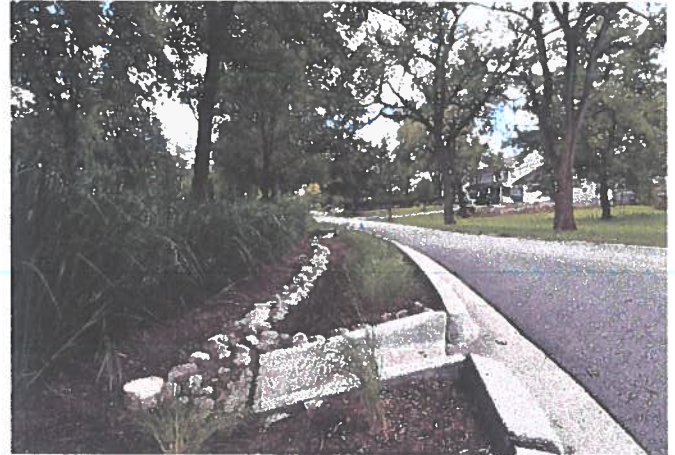
Curb cuts that drain to green infrastructure practices can be used as an alternative to traditional curbs and gutters.
