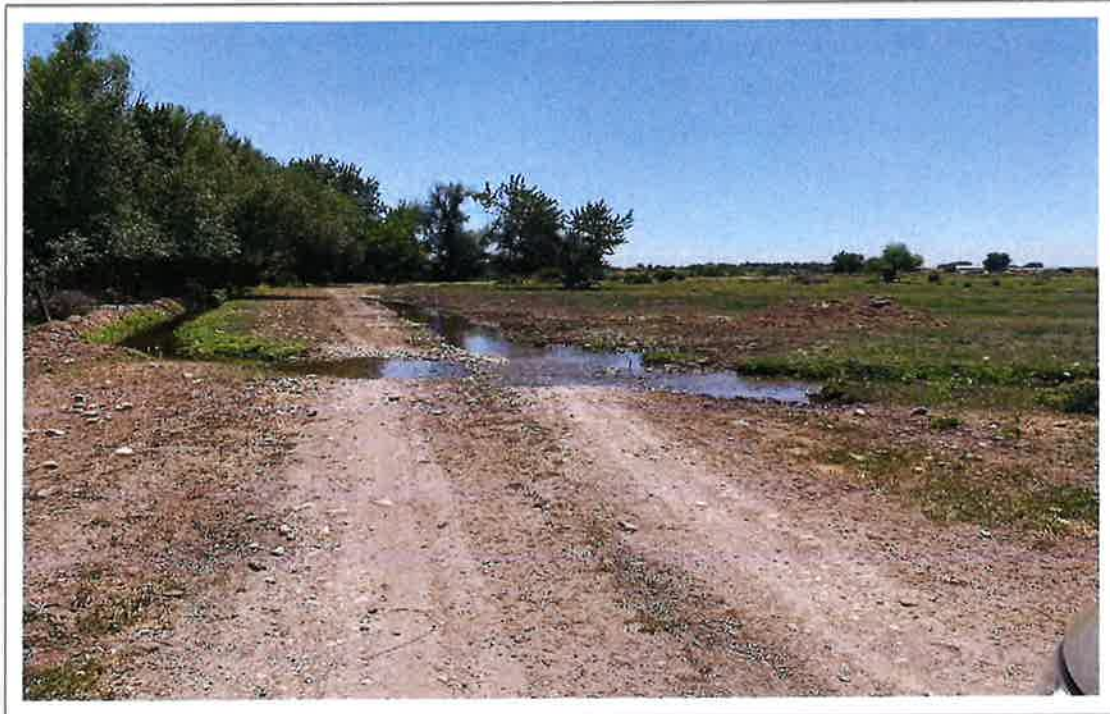
ACCESS ROAD SOUTH TOWARD HEADGATE SHOWING FLOOD IRRIGATION ACROSS ROADWAY.
