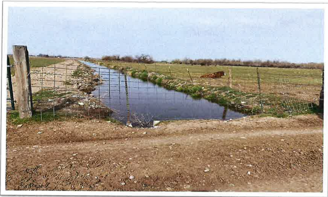
FRANKLIN DITCH (APRIL 2022) – WEST VIEW DEPICTING BOUNDARY BETWEEN NORTH AND SOUTH AREAS.
