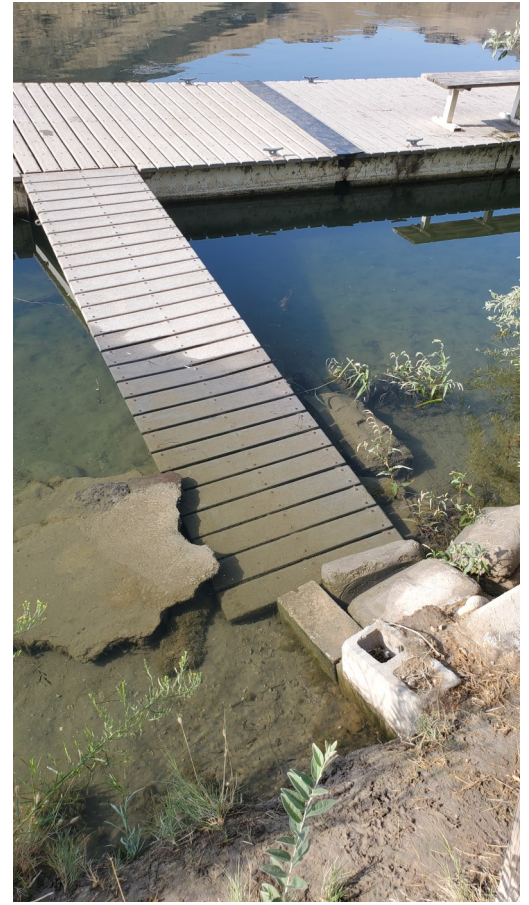
Above: our current dock system cannot adjust to changing river levels, leaving the gangways often underwater and inaccessible.
