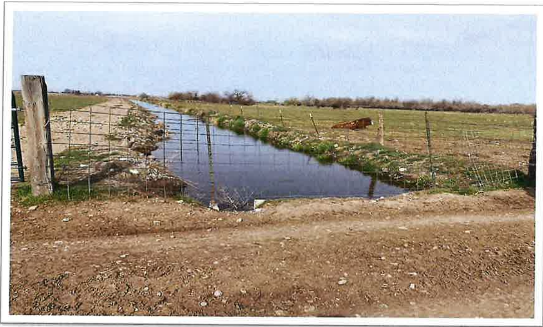
FRANKLIN DITCH (APRIL 2022) – WEST VIEW DEPICTING BOUNDARY BETWEEN NORTH AND SOUTH AREAS.
