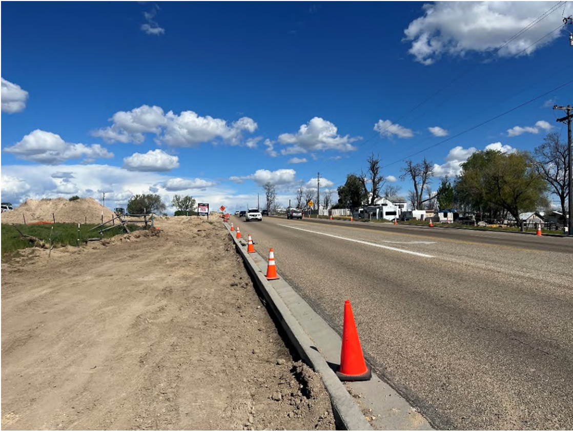
Looking East from access road down Amity Avenue.
