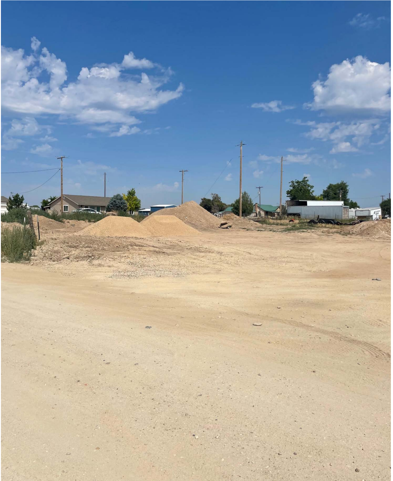
Image 5. Dirt staging area.
