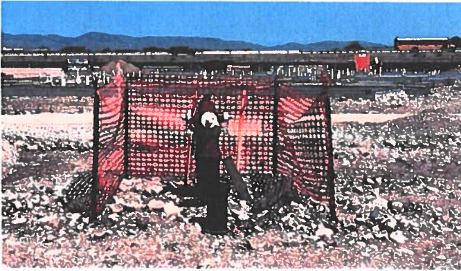
Hydrant marking during construction
