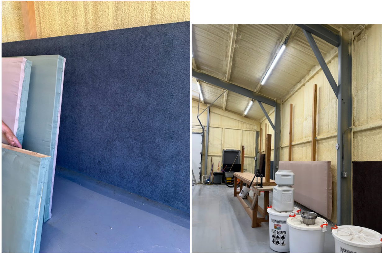
Figure 12. Foam and sound baffles to be installed to mitigate noise concerns.
