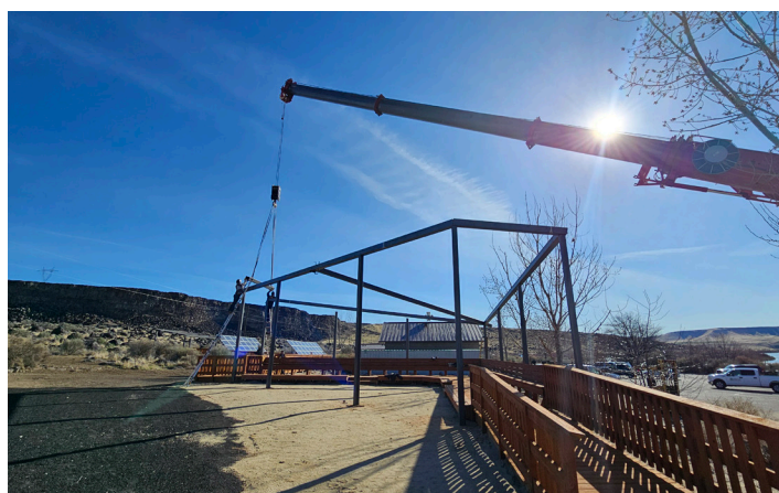
A crane lifts the shade-structure beams into place.
