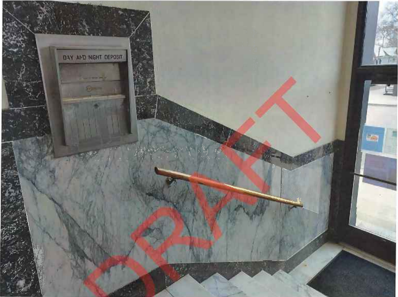
Photo 11 of 24. ID_Canyon_ParmaStateBank_0011 View of vestibule interior and night deposit box, camera facing northeast
